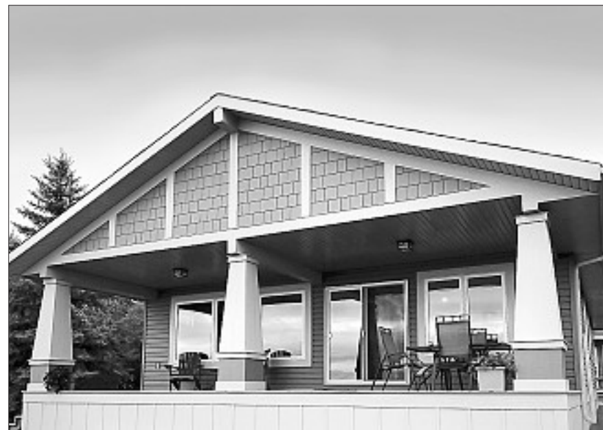
There's nothing left for buyers to do at Waters Edge but move in, the developers say. "We completely landscape the lot ...," says Rick Arndt, a project founder. "We put a firepit in the front yard, the deck is built, sidewalks are on."
